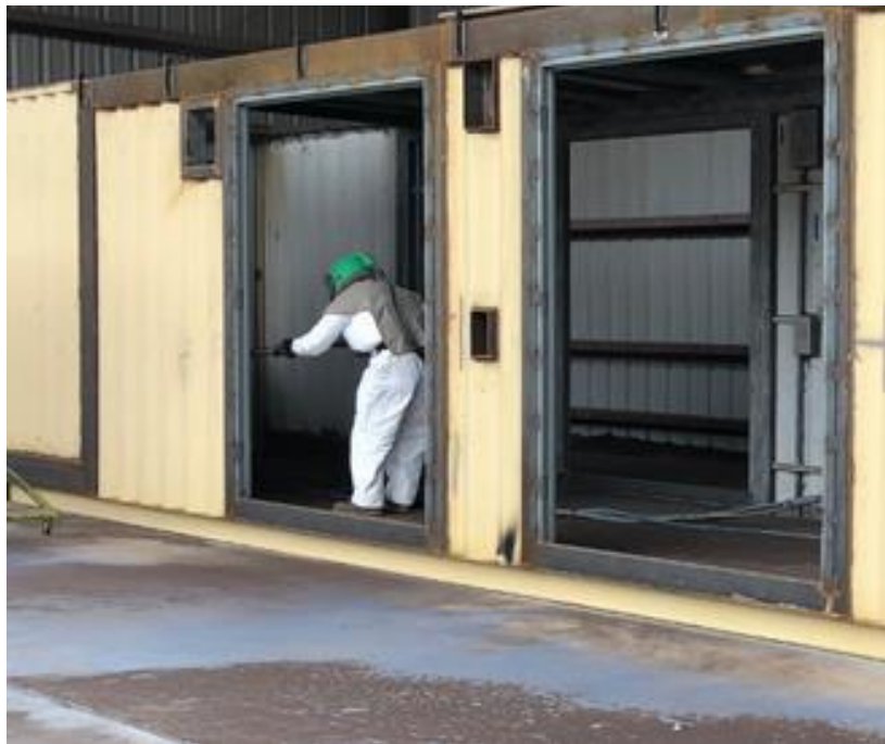
Figure 4-2 – Container blasting prior to painting
