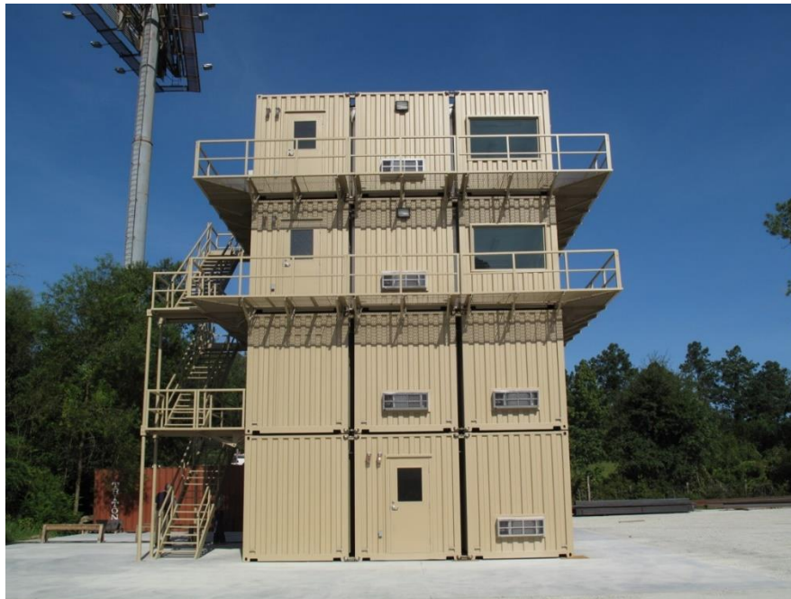
Figure 5-9, Example of past Jenshau work
