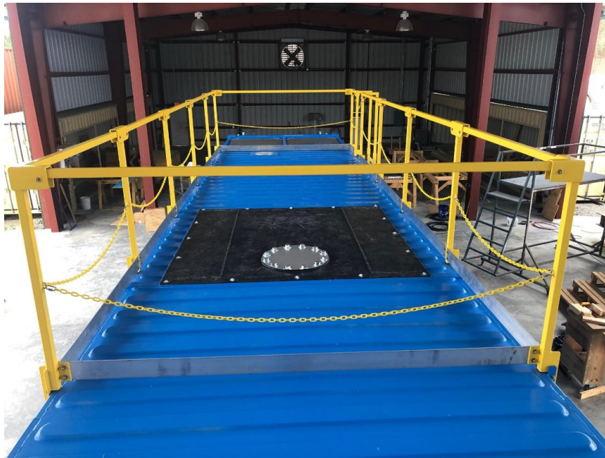
Figure 5-8, Design build ladder and railing system
