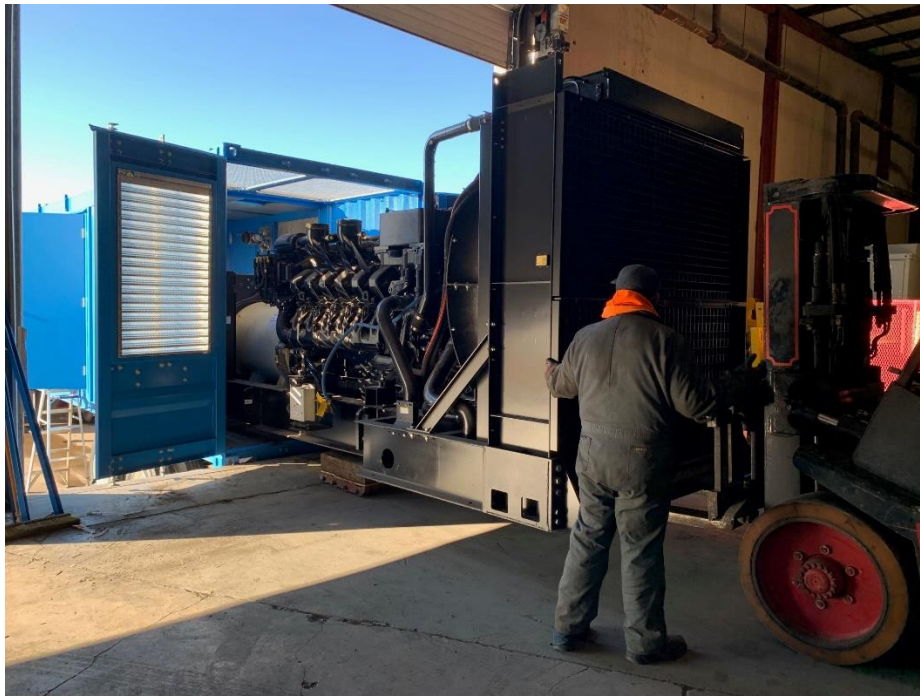
Figure 5-14, Example of past Jenshau work
