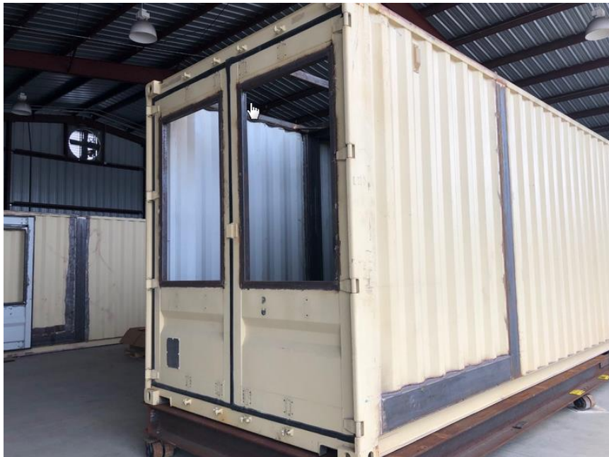
Figure 5-6, Example of container modification – roof, sidewall and doors
