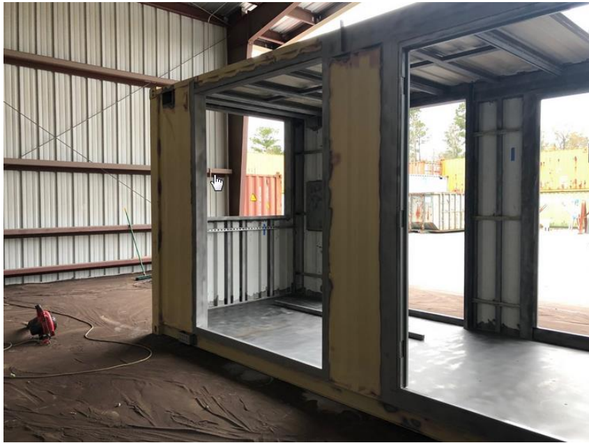
1. Figure 4-3 – Container blasting prior to painting
