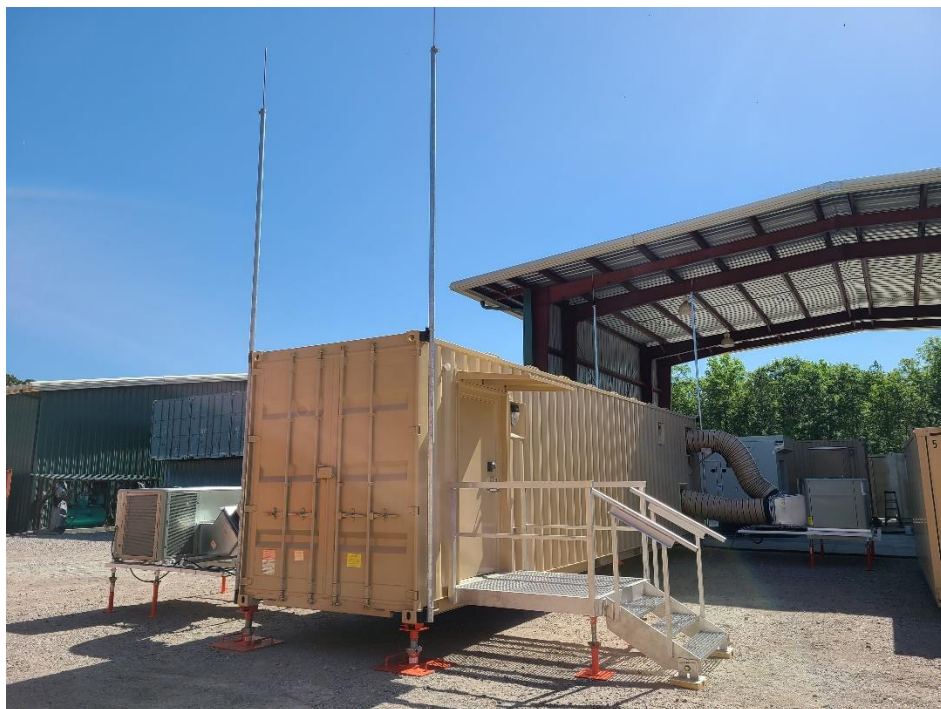
Figure 5-17, Example of past Jenshau work
