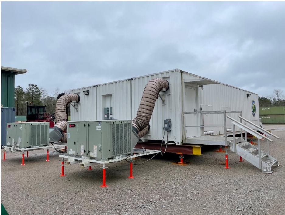
Figure 5-12, Example of past Jenshau work
