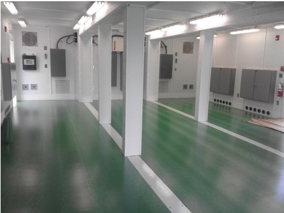
Figure 5-13, Example of past Jenshau work
