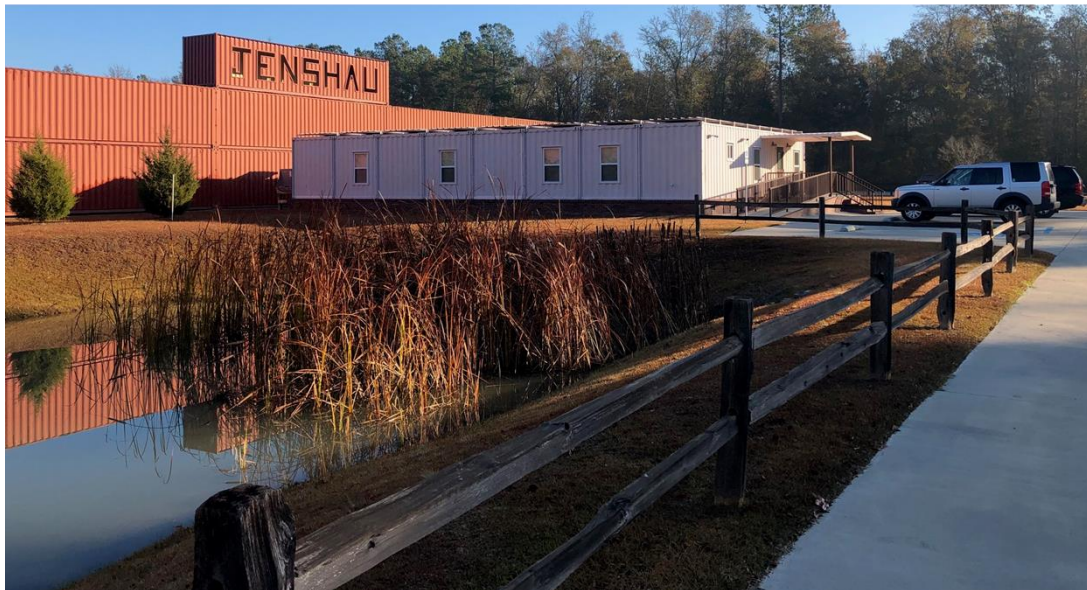
Figure 1-3, Jenschau office facility.
