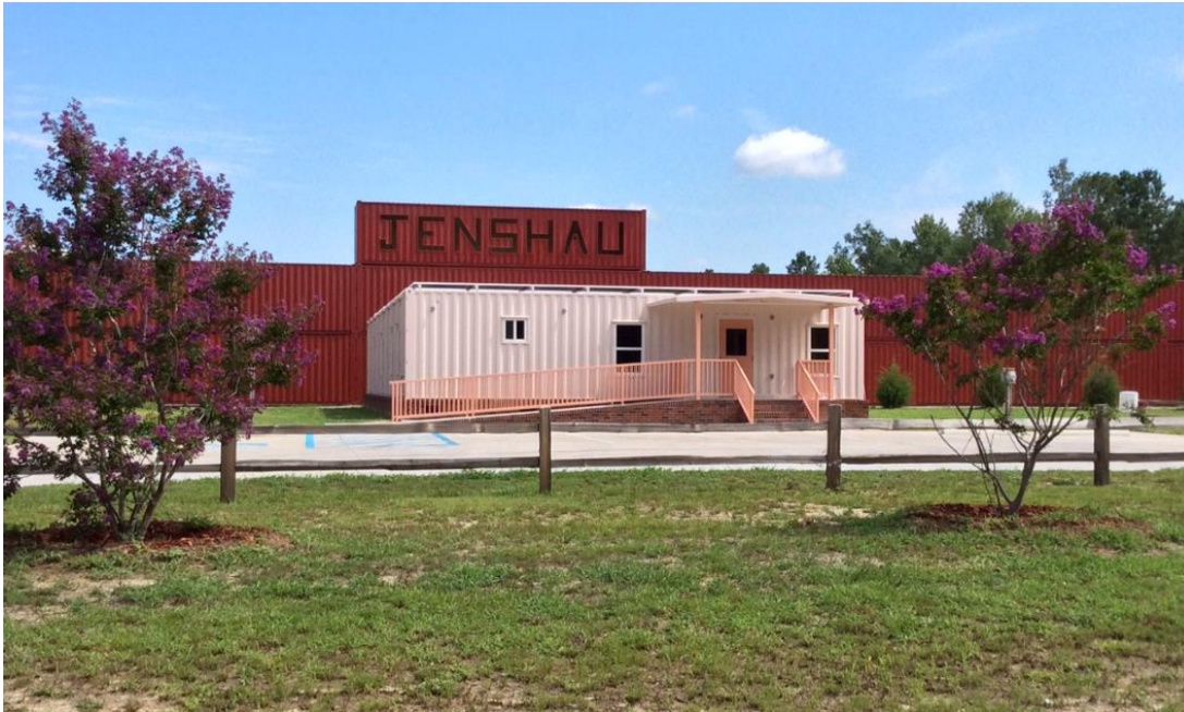
Figure 1-2, Jenschau office facility
