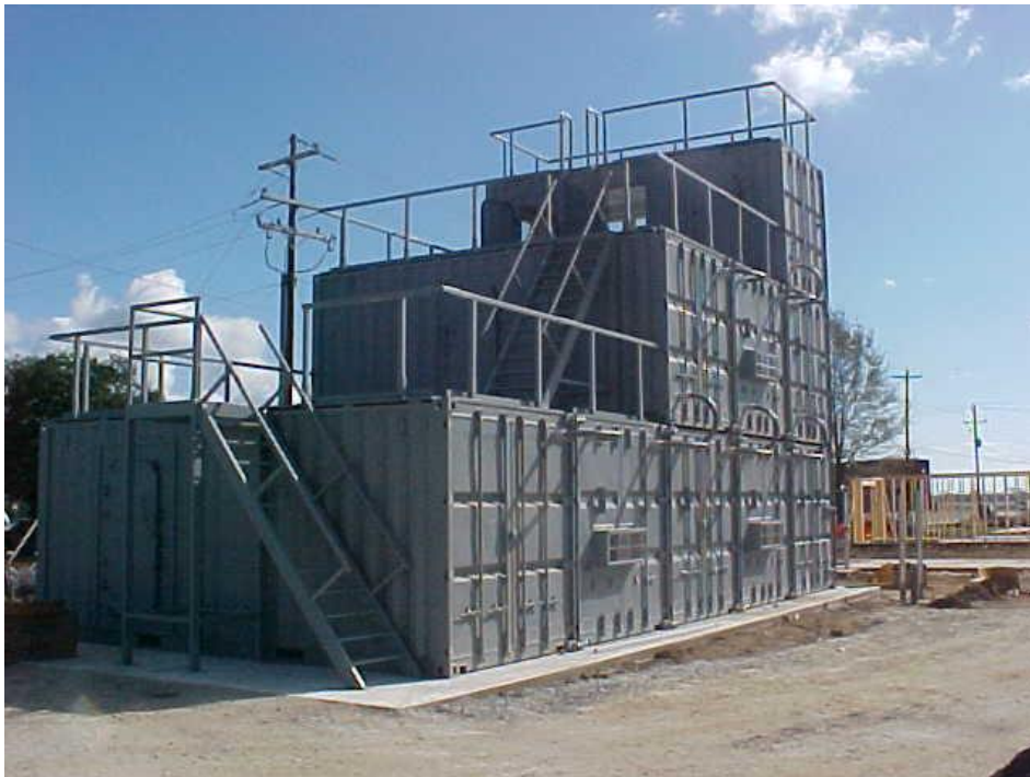
Figure 5-16, Example of past Jenshau work
